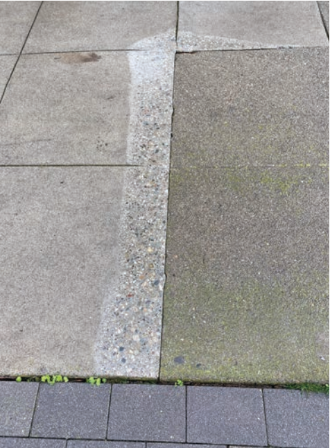
San Francisco Public Works pays for sidewalk grinding throughout the City. The measure is supposed to even out pathways and protect against tree root disruption. Often times the grinding takes place adjacent to significant bumps, cracks, and divots, which are left unremediated. PHOTO: Potrero View Staff
