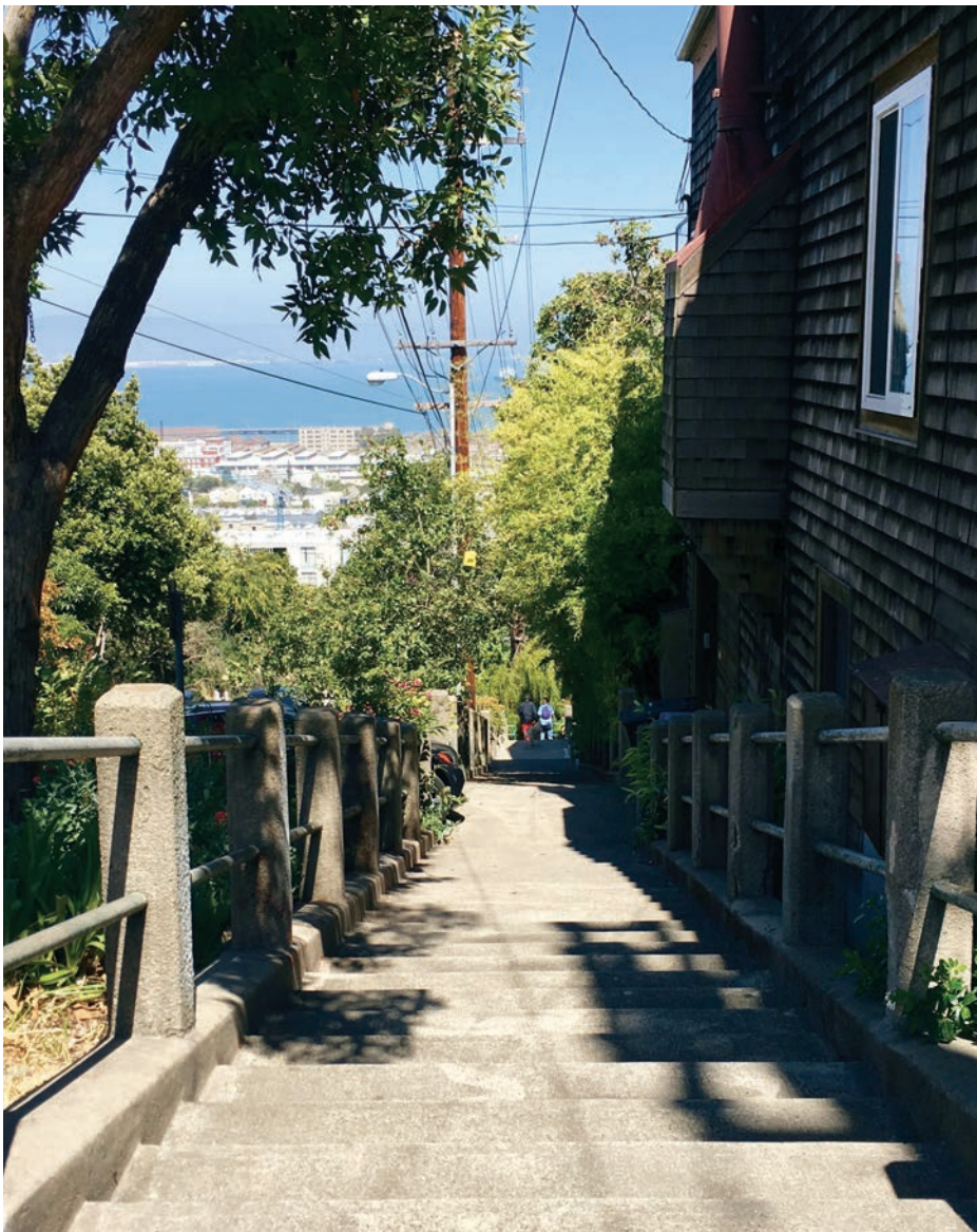
A staircase at 22nd and Wisconsin streets.
