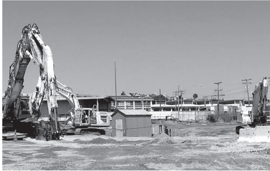
Potrero Power Plant remediation work in progress.
