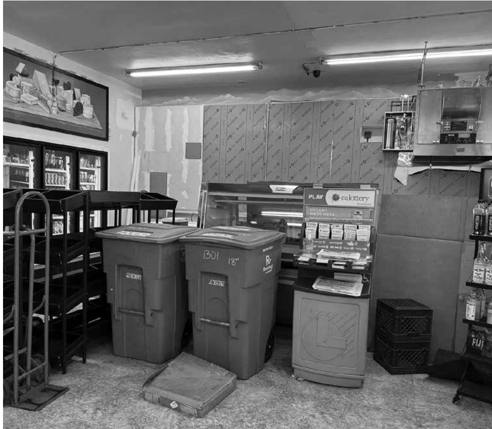
New Potrero Market under renovations. PHOTO: Mike Lin
